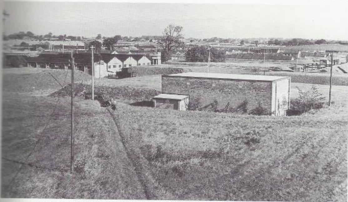
Looking north from Pump House No. 2, a photograph which shows nicely the earth 'traverses' or blast banks which separated the buildings within the factory. The idea was that in the event of an accident in one building, the blast would be diverted upwards and should not affect adjacent buildings. The vehicle in the middle foreground was the photographer's van.
